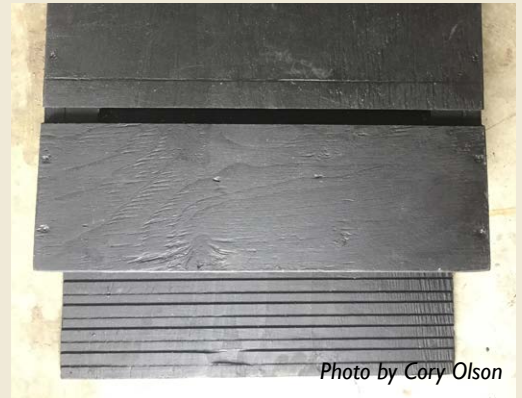
Bat houses need at least a 4" landing strip so bats can land and crawl inside.
