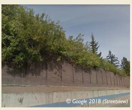
Acoustic walls are often used along busy roads to reduce sound emissions to neighbouring communities. Mobile sound barriers are also available to dampen emissions from industrial facilities, such as compressor stations and drilling rigs. These technologies may help reduce the effects of sound on the quality of bat foraging habitat.
