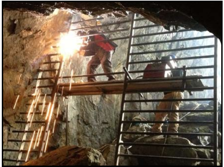
Lower Adit gate being constructed on Queen Victoria mine.
